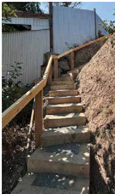
Newly completed Weir Beach access stairs with handrail. J. Shukin photo
